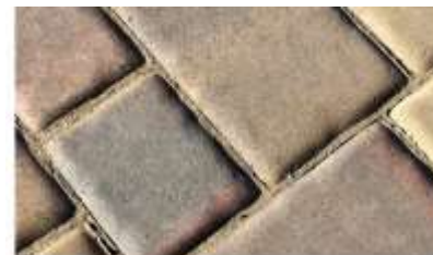
Worn DuraFusion Pavers
